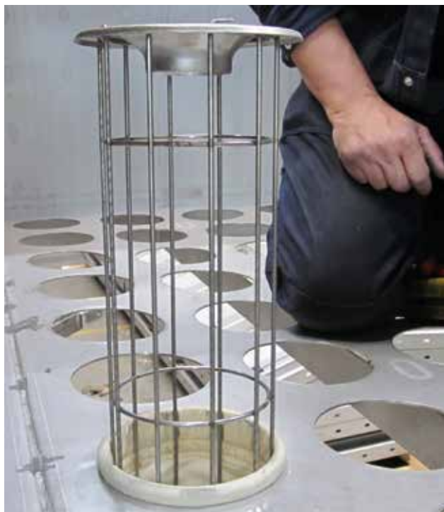
Support cage in filter bag
